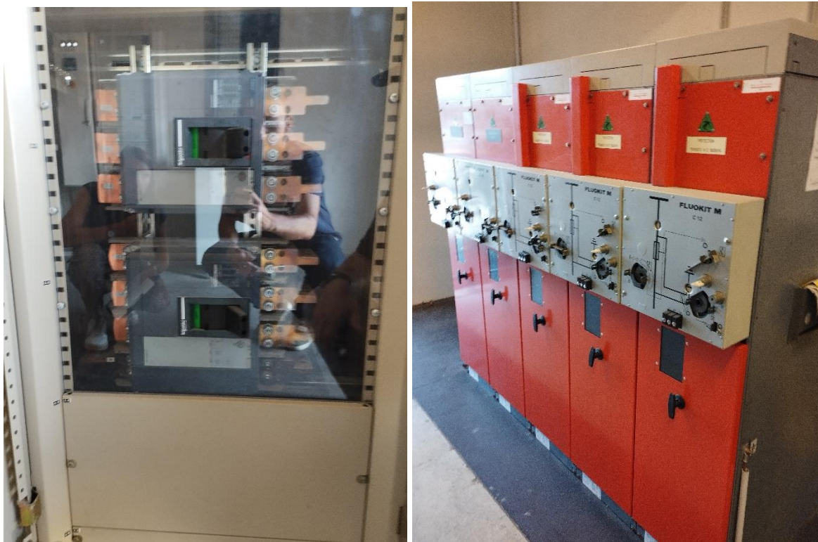
Figure 28 Poste de transformation T - Raccordement BT zone 2
