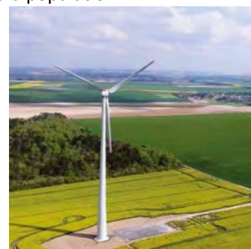
Eolienne terrestre © wpd
