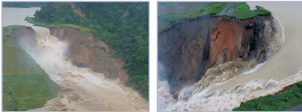
Figure 8.139 Failure of the El Guapo Dam, Venezuela, December 1999 (courtesy M Morris)
