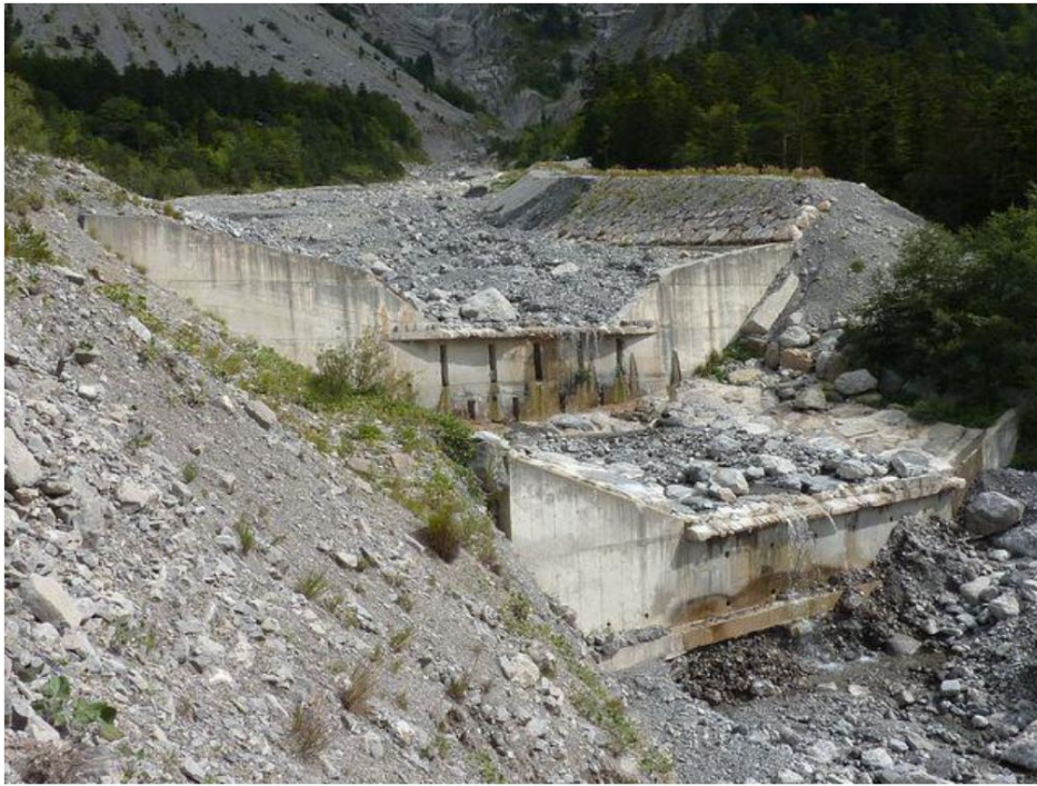
Figure 9 : Barrage Lombard B2 (JBN, service RTM, 2010)
