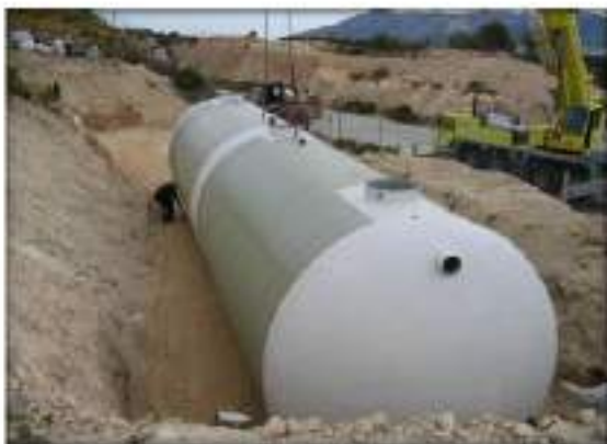
Pose Station Type BIOXY FIX
