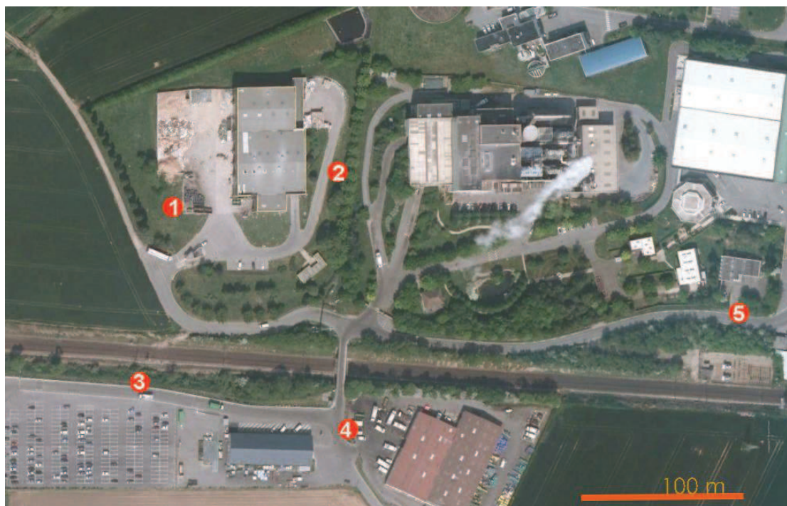
Figure 119. Localisation des poteaux incendie
