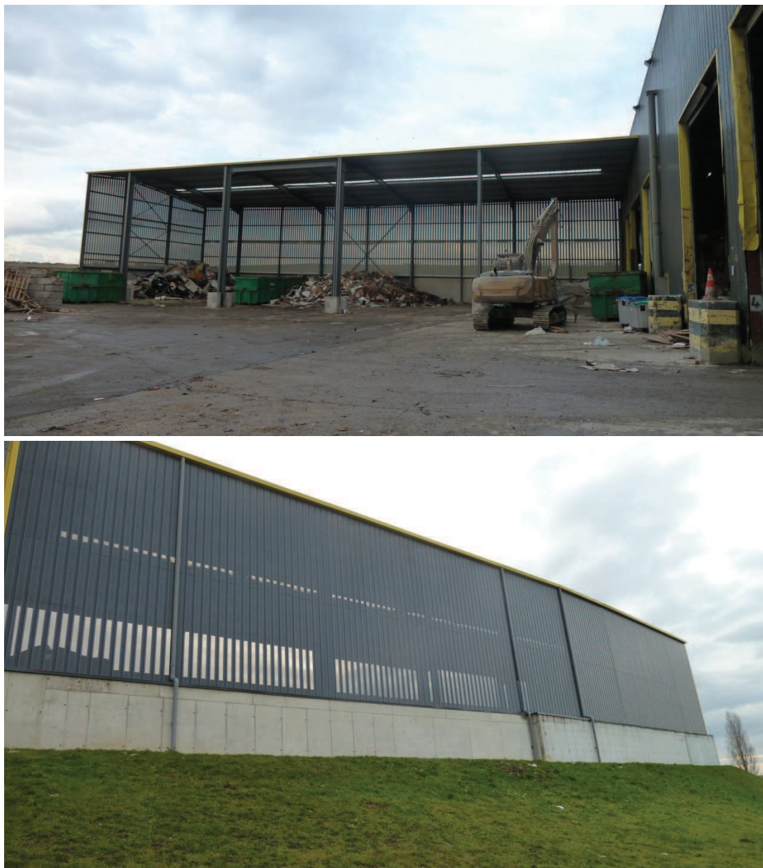
Figure 34. Photographies abri couvert
