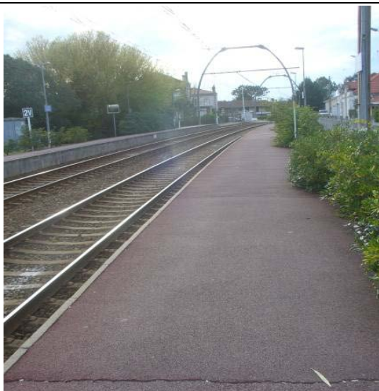
Photo 13 – Quai n°2 direction Arcachon
