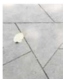
Joints de dilatation
