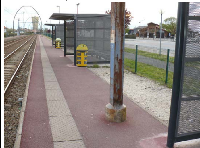
Photo 13 – Quai n°2 - direction Arcachon
