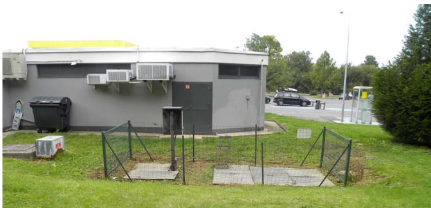
Station d'épuration de la station service
