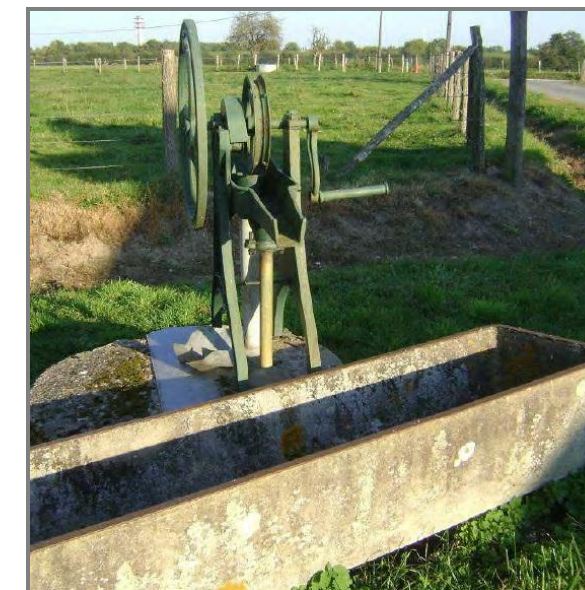
Figure 25 : Captage AEP privé (Source GENIVAR)
