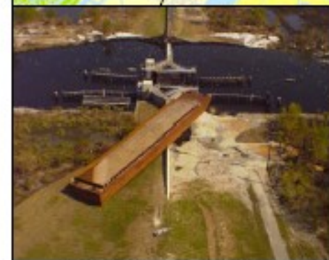
Bayou Bienvenue Control Structure
