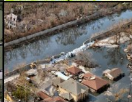
Canal Breach at Mirabeau
