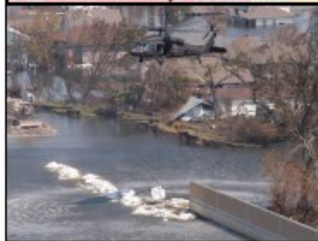
17th St. Canal I-wall Breach
