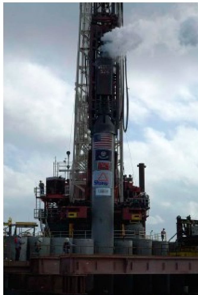
Last Pile Driven Oct 23, 2009
