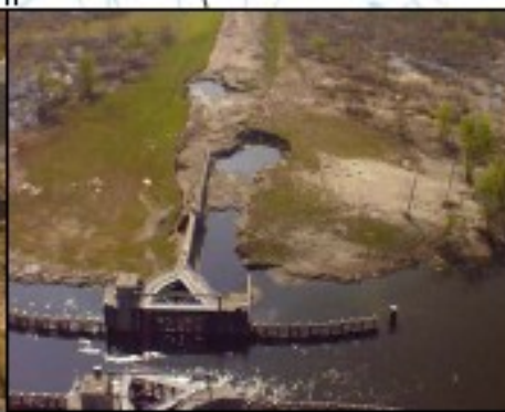
Bayou Dupre Control Structure
