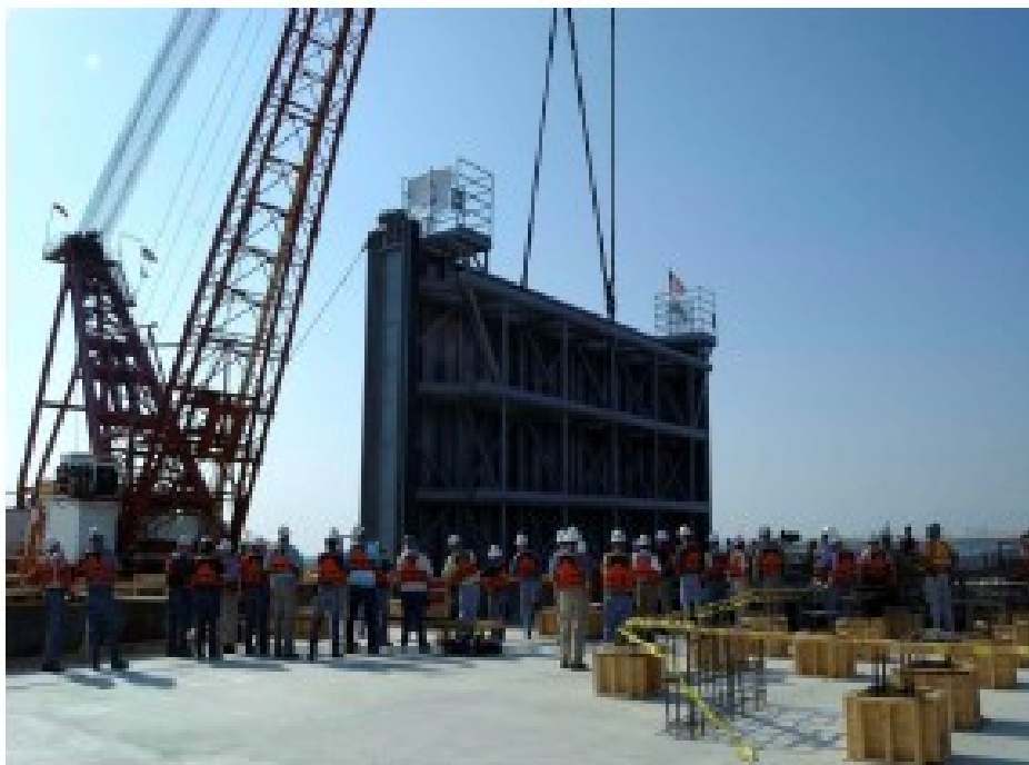
Bayou Bienvenue Gate Installation
