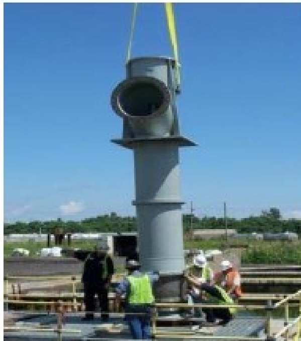
Repair 61 pump stations ($103 Mil)
