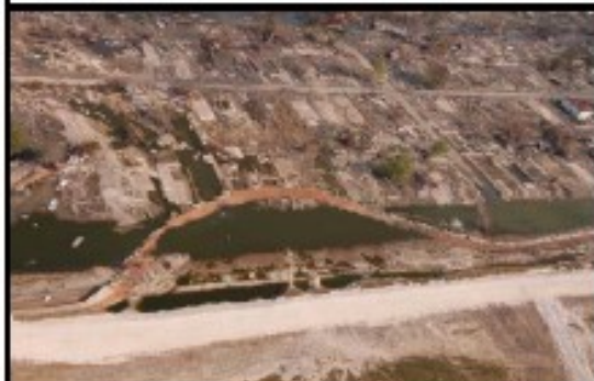
Sheetpile Floodwall Collapse
