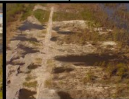
Intracoastal Waterway Breach
