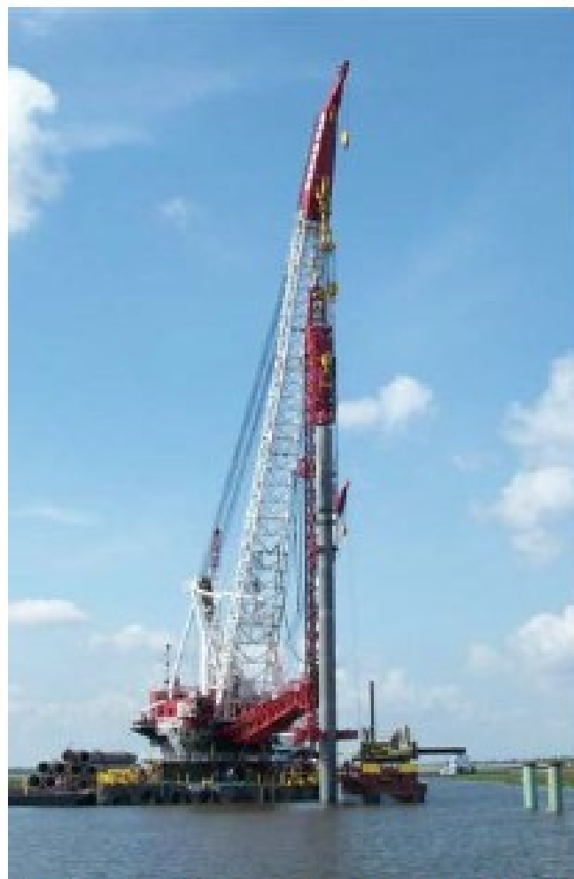
First Pile Driven May 9, 2009
