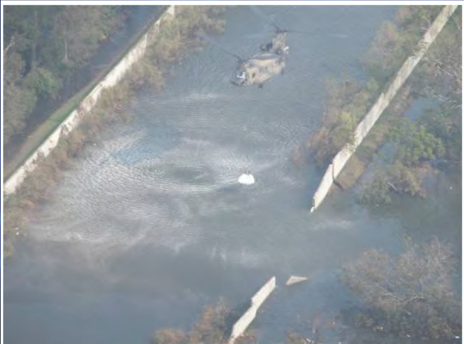
Figure 28. South Breach, London Avenue Canal
