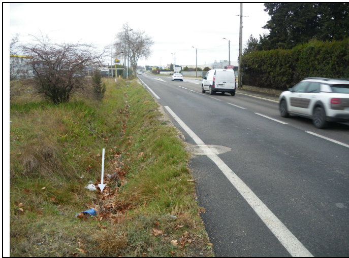
Photo 1 : Fossé pluvial RN 580
