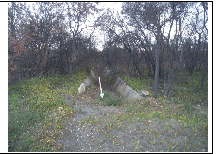
Photo 8 : Canal béton amont FM Logistic
