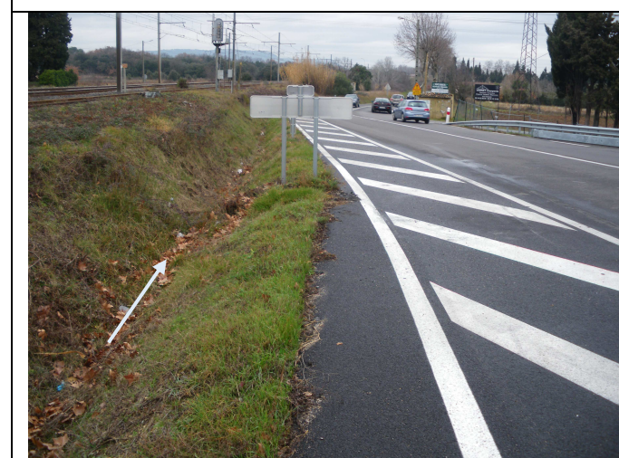
Photo 11 : Fossé pluvial RN 580
